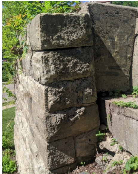
Figure 3. Example of failure along east side of the existing structure (note the gap between the concrete slabs and multiple generations of repairs)
