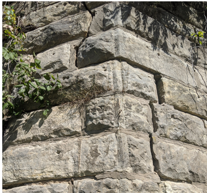
Figure 7. Distress along the southeast corner of the existing structure (note the shifting of the east wall, mortar repairs made, and cracking through blocks)
