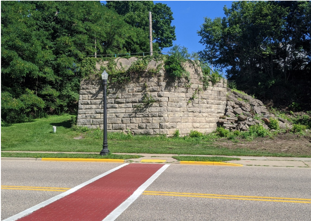
Figure 1. Former bridge abutment for Oak Street looking north from Water Street (note the slope failure along the east side of structure)
