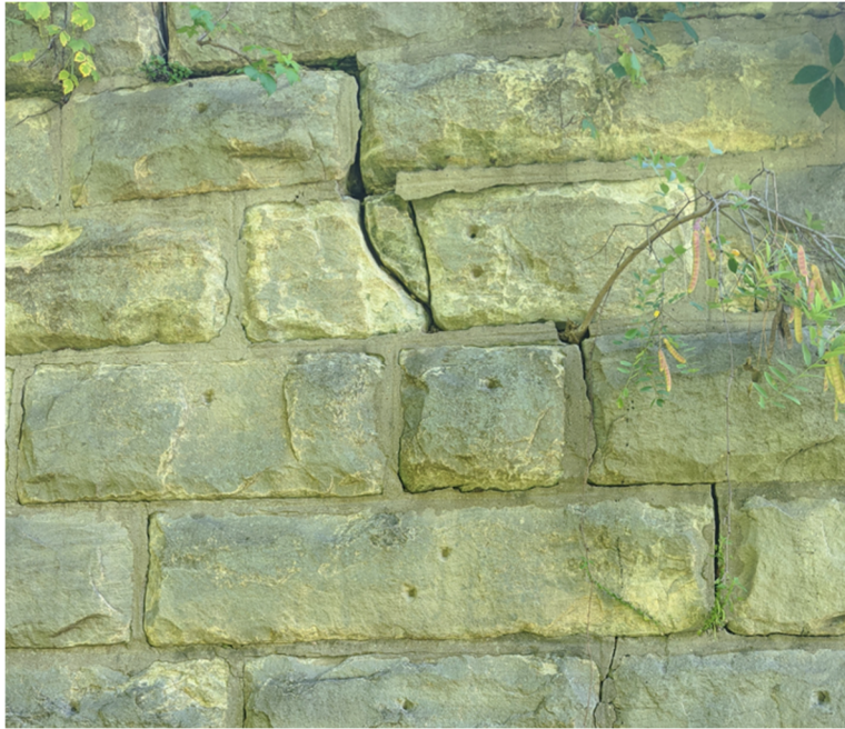
Figure 6. Distress and shifting of the existing structure resulting in voids and failure along the west wall
