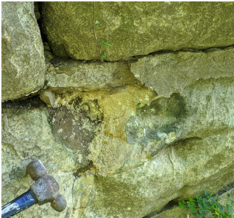
Figure 9. Existing stone has weathered and is not structurally sound for a retaining wall of this height. Reuse of the stone for smaller walls, planters, or decorative outcroppings is recommended.
