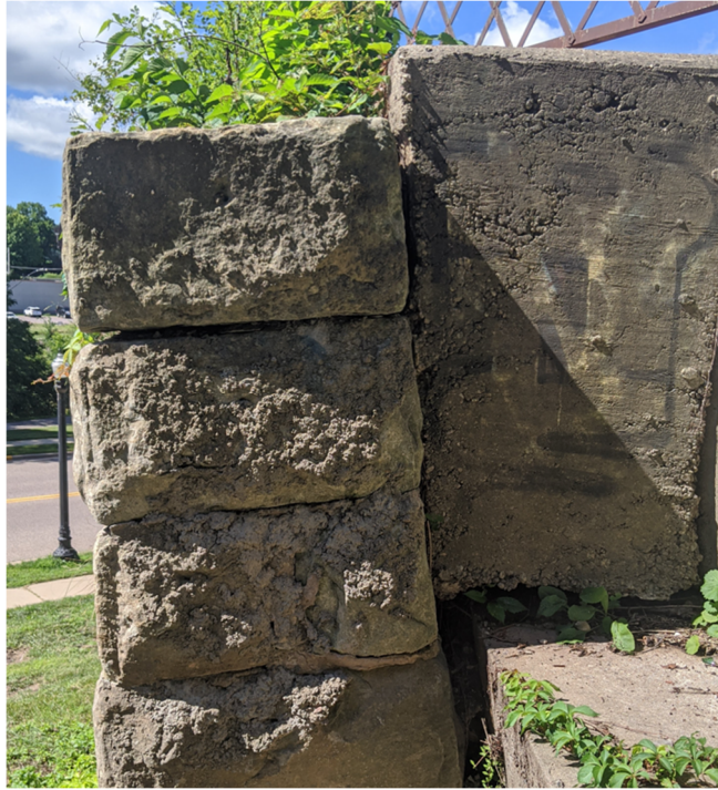
Figure 8. East wall has shifted and is beginning to fail near the top of the structure
