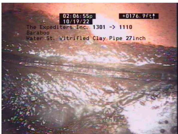
1301-1110_4f2f81b9-6de3-464a-8883-a2f8e97a7e85_20221019_141714_789.jpg, 00:06:13, 176.90ft Infiltration Runner Joint from 7 o'clock to 11 o'clock, within 8
