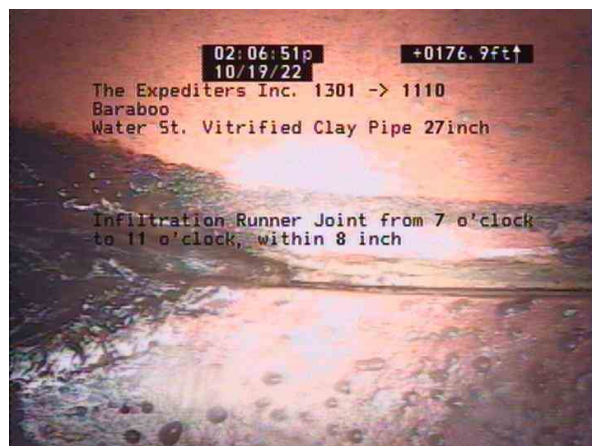
1301-1110_c7d9c086-119b-421f-89a7-bedb0ce2f169_20221019_141710_746.jpg, 00:06:13, 176.90ft Infiltration Runner Joint from 7 o'clock to 11 o'clock, within 8
