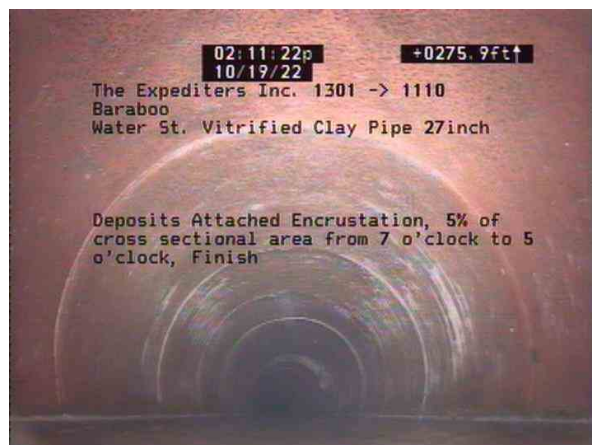
1301-1110_c5cbc2eb-4fed-4bfa-a26f-fbb0eb412954_20221019_142141_995.jpg, 00:10:11, 275.90ft Deposits Attached Encrustation, 5% of cross sectional area from 7 o'clock to 5 o'clock, Finish
