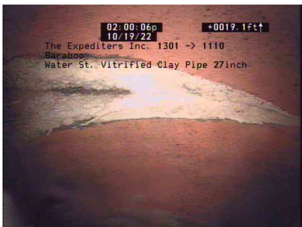
1301-1110_27281dfa-0887-4f94-b4b3-f6e918ad30df_20221019_141025_887.jpg, 00:00:50, 19.10ft Deposits Attached Encrustation, 5% of cross sectional area
