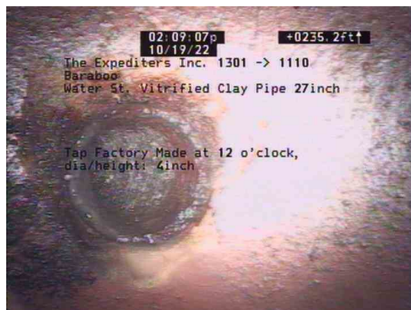
1301-1110_67812f3f-5799-46fc-91ef-65eb56d35a24_20221019_141926_751.jpg, 00:08:22, 235.20ft Tap Factory Made at 12 o'clock, dia/height: 4inch
